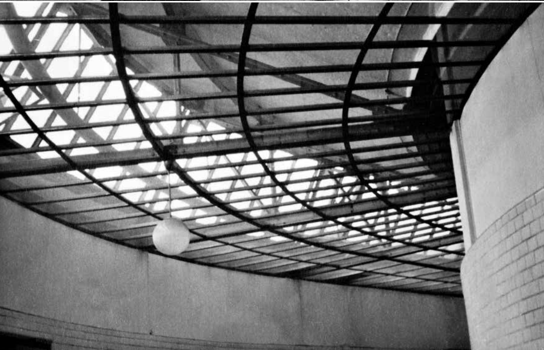
Dessau Employment Office, glass panels being reinstalled after cleaning, 1955
